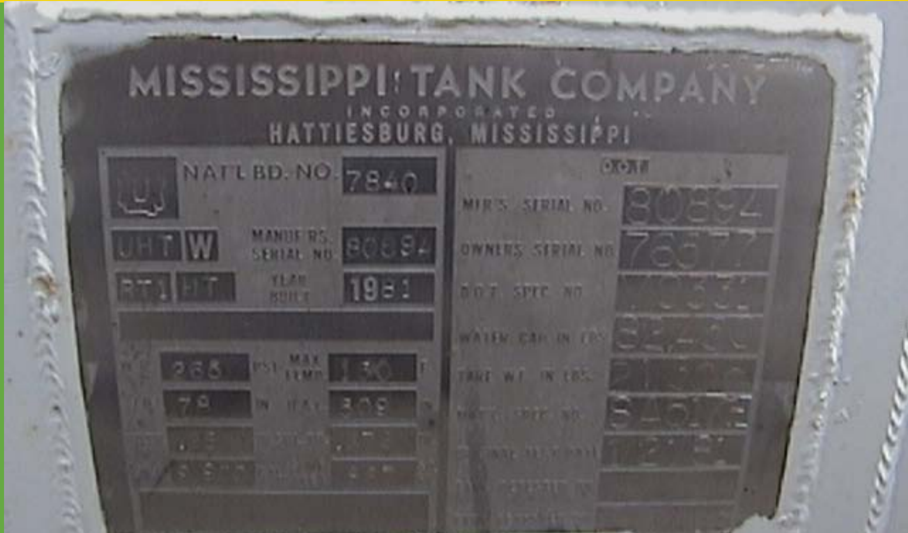
MANUFACTURER'S DATA PLATE FOR LPG STORAGE TANK
